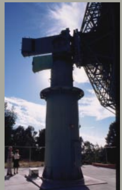
Researchers Manfred Bester and Nahide Craig of the UC Berkeley Space Sciences Laboratory are dwarfed by the antenna used to track RHESSI and other satellites.
